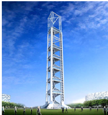
Fig. 4 Single Truss in Beijing, Transmission Tower.
